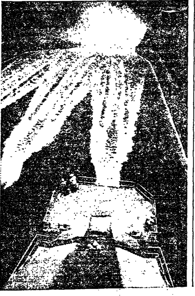
The Itaipu dam, on the Parana river that forms the border between Paraguay and Brazil, is the largest hydroelectric development in the world. When the 18 turbines finally come on stream in 1983 it will generate 12,600 megawatts of electricity, six times the power of Egypt's Aswan dam.
